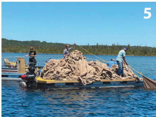
5. Beginning deployment of barrier. The yellow line to the left is 600 feet long and runs over the center of the EWM bed. It is attached to a large anchor. As we pull on this line, the barrier runs off the boat, pausing at intervals to set side anchors.
