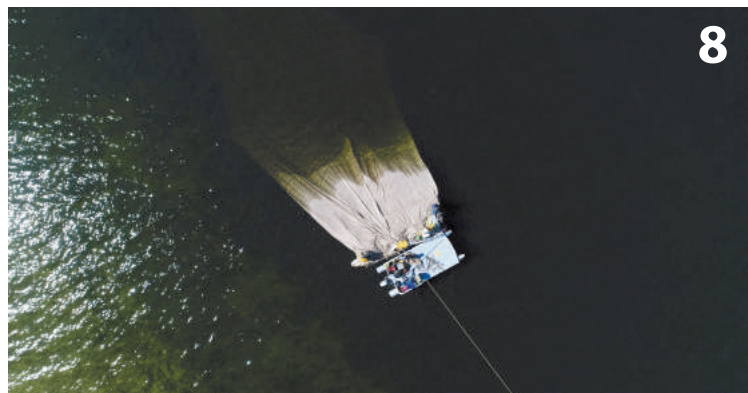
7. Drone shot of barrier being deployed off the shoal adjacent the Mebert Creek Natural Area in Bingham Township. In all, 1,400 feet of barriers now cover continuous Eurasian Water Milfoil that has been established on the drop-off north of Gordon's Point.
